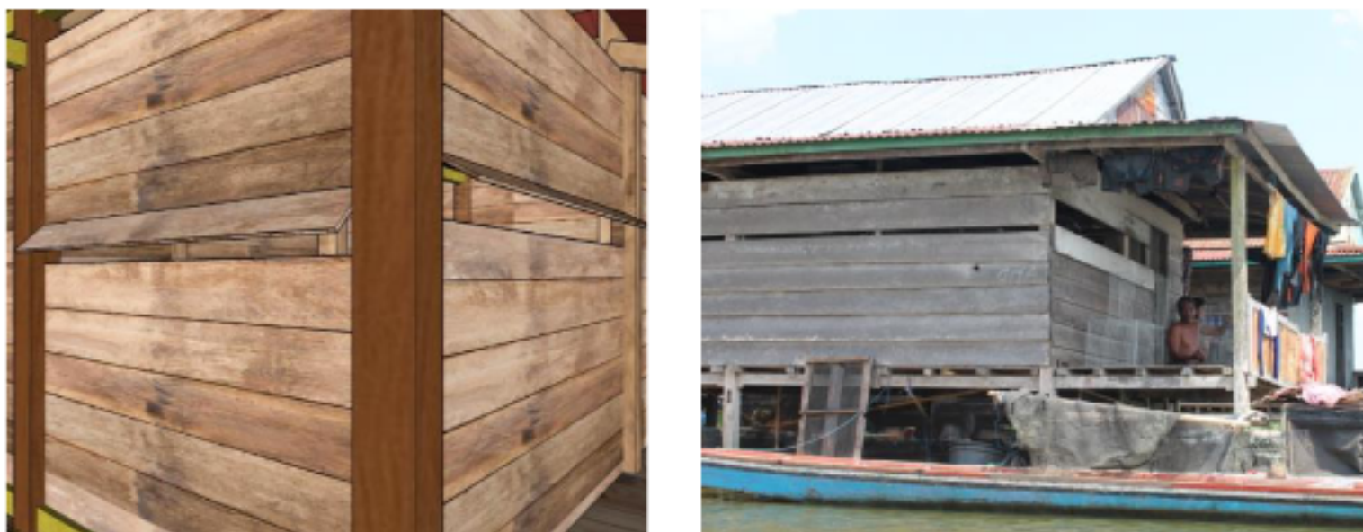
Figure 9. Type 2 Board Wall Construction Details on the Front and Side Source: Personal Photos & Sketches, 2021
