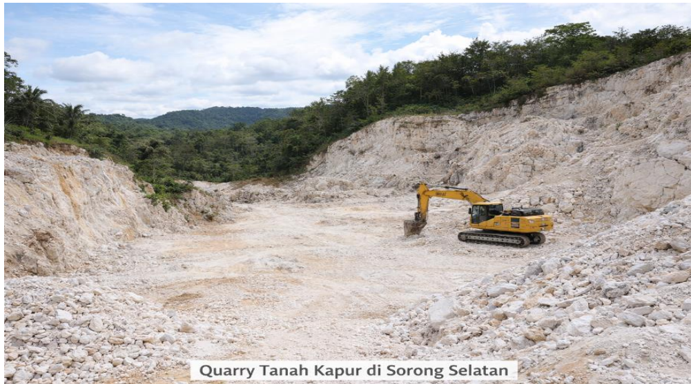
Gambar 3.2 Lokasi Pengambilan Material (Quary)
