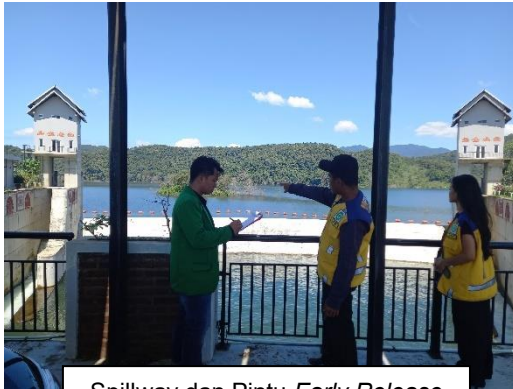
Spillway dan Pintu Early Release
