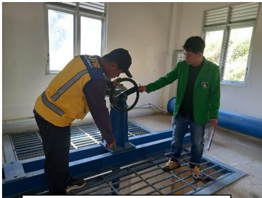
Aktuator Hollow Cone Valve
