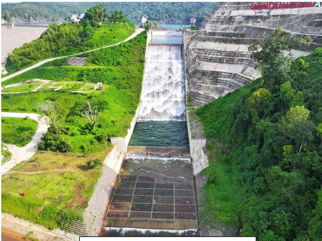
View Downstream Bangunan Pelimpah/ Spillway
