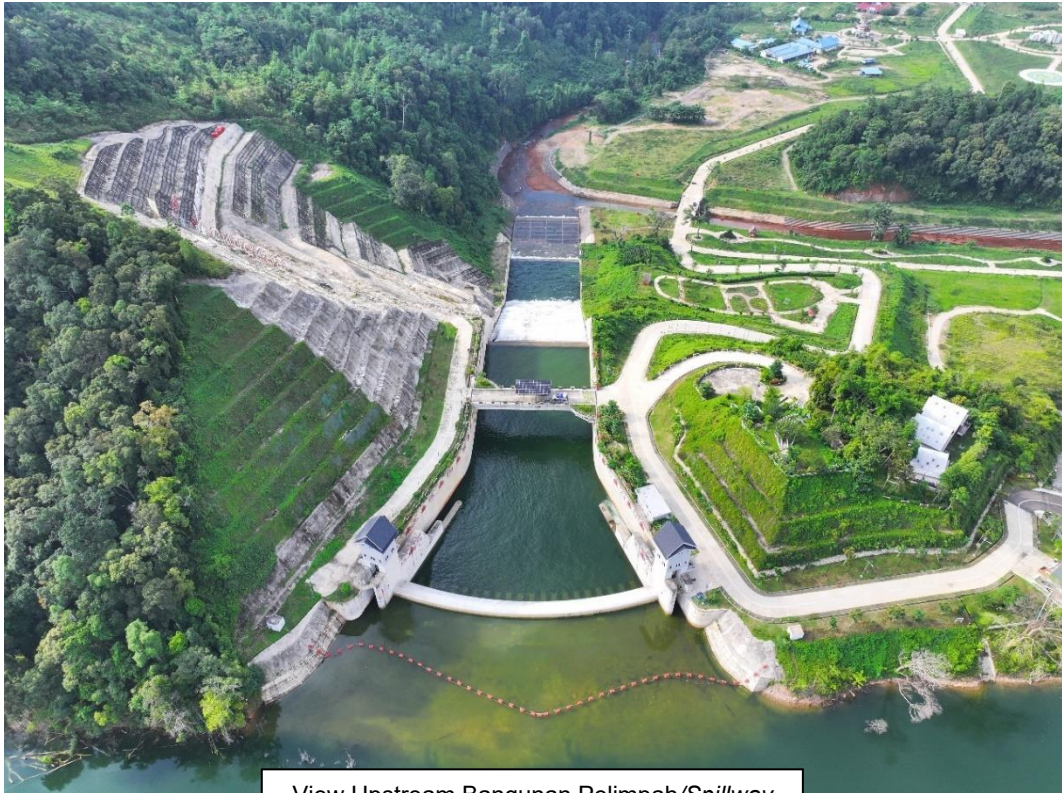
View Upstream Bangunan Pelimpah/ Spillway
