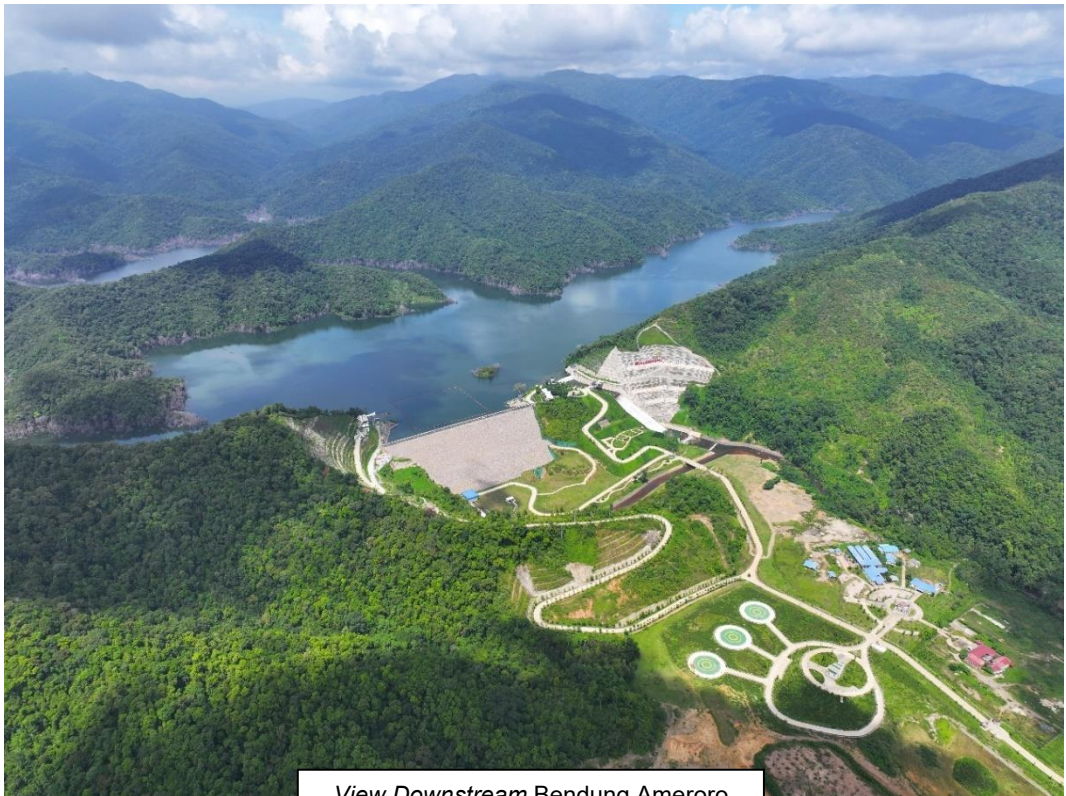
View Downstream Bendung Ameroro
