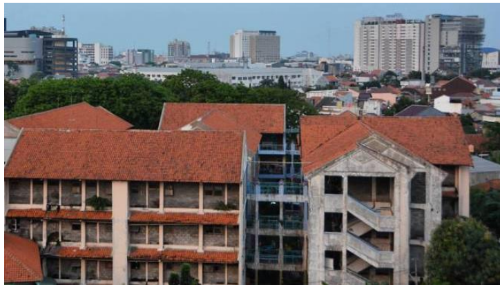
Figure 2. Condition of Pekunden Flat (www.google.com)
