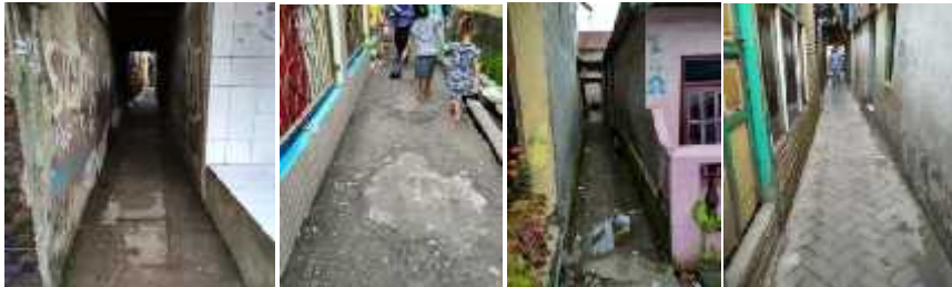
Figure 9. Physical condition of street
