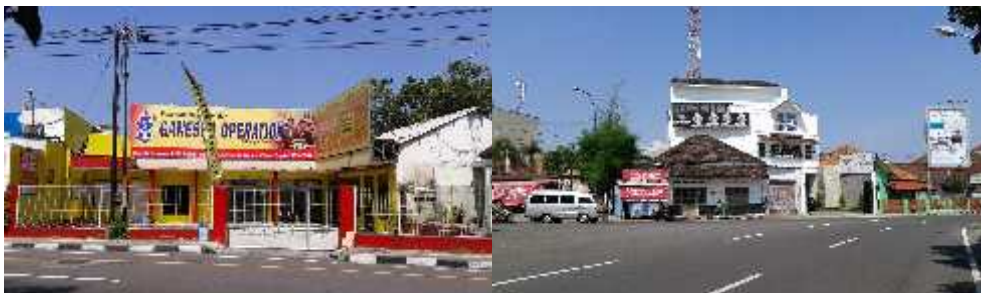
Figure 18. New buildings which are not contextual to their surroundings Source: Survey, 2017
