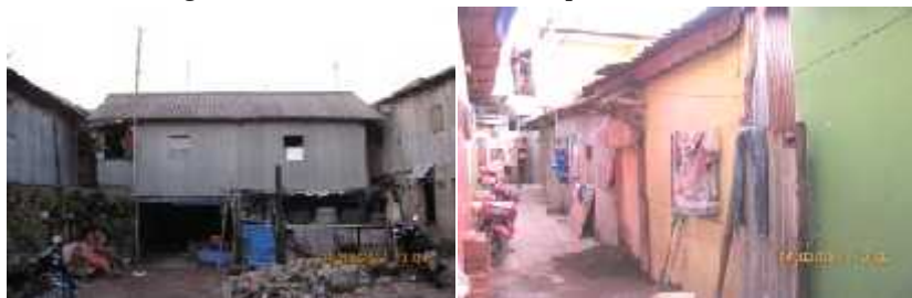
Figure 6. Physical condition of housing
