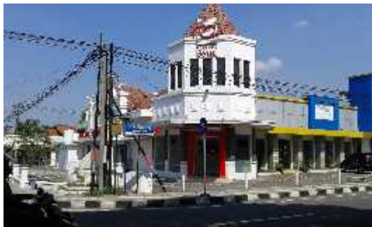
Figure 16. The old building which is modified and changed into a new function Source: Survey, 2017
