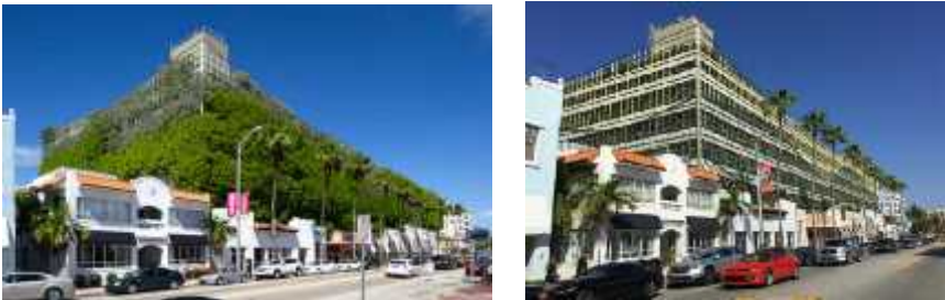
Fig1: Vertical Green Application on Urban Corridor Source: Pinterest (2017)
