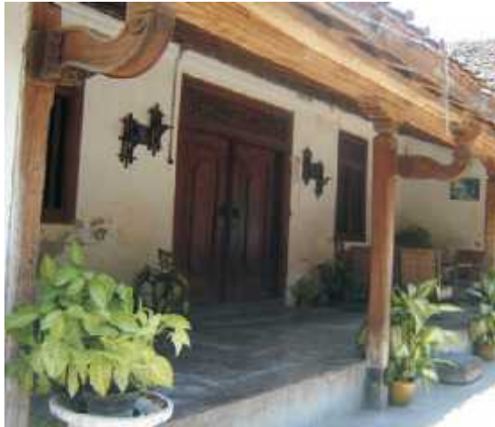
Figure 9. Bahu dhanyang, which supports the overhang, has an aesthetic function.
