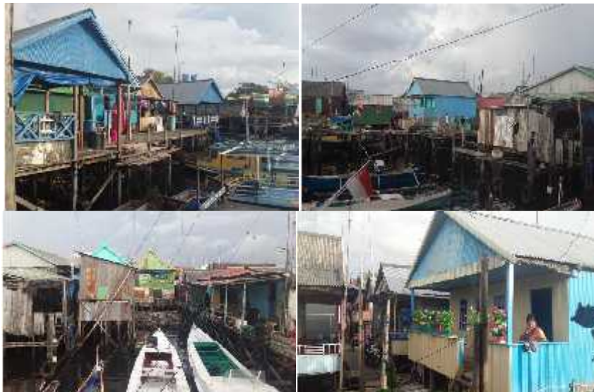
Figure 3 (Continuance). Physical Building Condition in Zone 1
