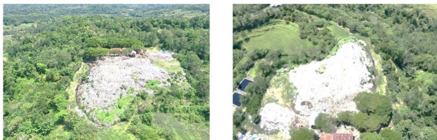
Figure 5. The condition of the Tondong FDS
