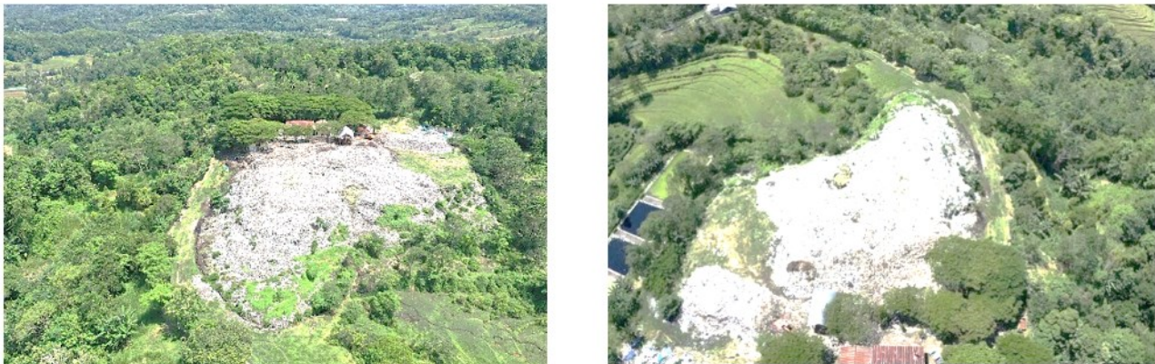
Figure 5. The condition of the Tondong FDS
